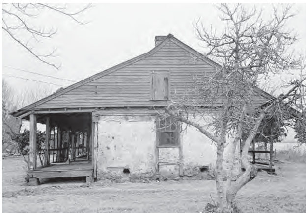
Figure 6-1. East side of La Pointe-Krebs House in 1936.
