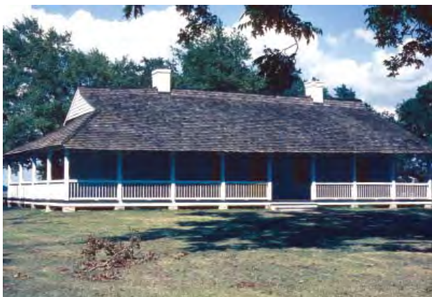
Figure 1-13. La Pointe-Krebs House after the 1995 restoration.
