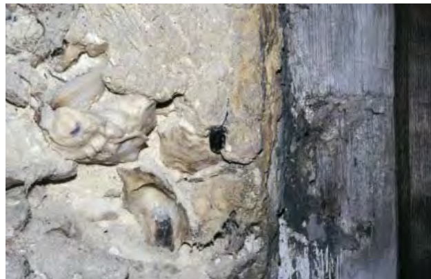
Figure 6-8. Tabby in-filled wall of La Pointe-Krebs House.
