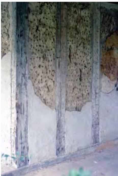
Figure 6-7. Plaster-covered bousillage in-filled wall of La Pointe-Krebs House.
