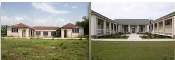
The Randolph School in Pass Christian before and after rehabilitation
