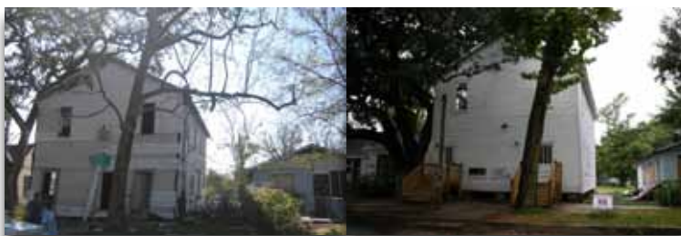
The Rectitude Masonic Lodge in Gulfport before and after rehabilitation
