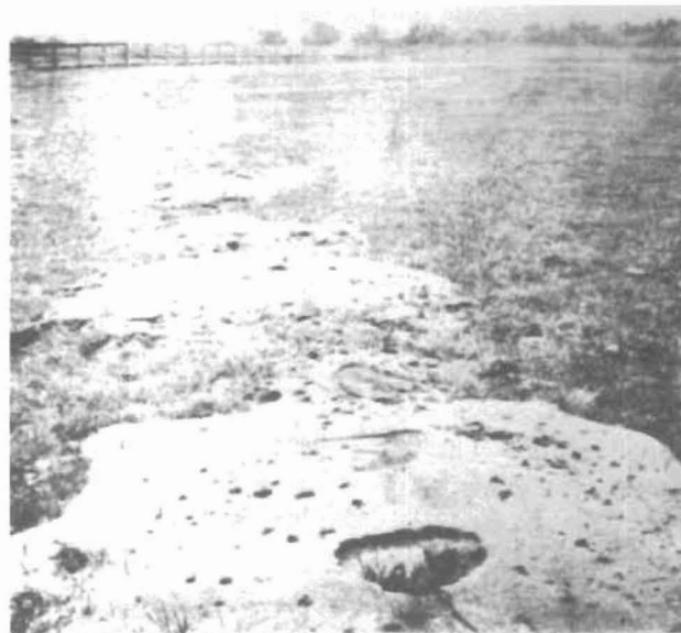
SAN FRANCISCO, CALIF EARTHQUAKE OF 1906
